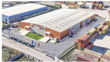
Warehouse in Thessaloniki - Greece
