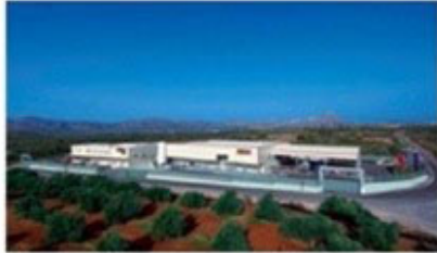
Central facilities – Factory in Chania – Crete- Greece
